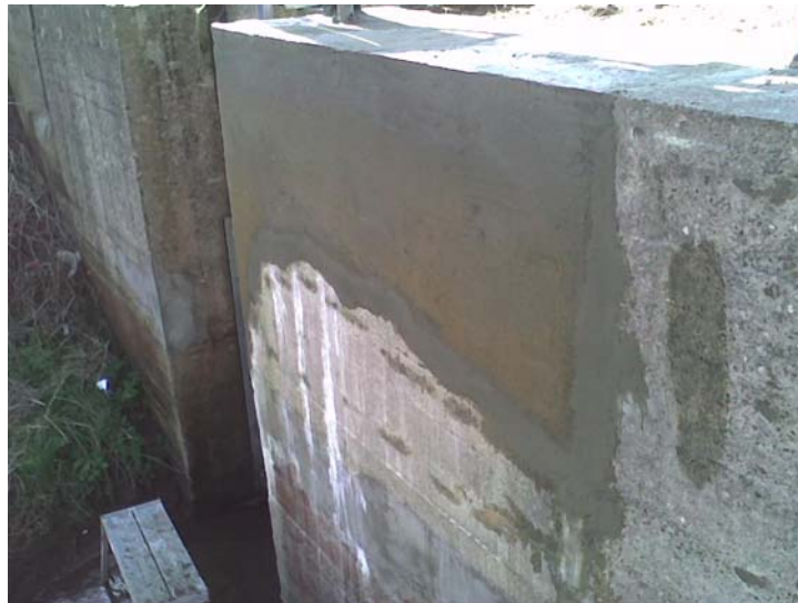
Concrete Repairs to the freeze thaw damage at Fosdyke Sluice
